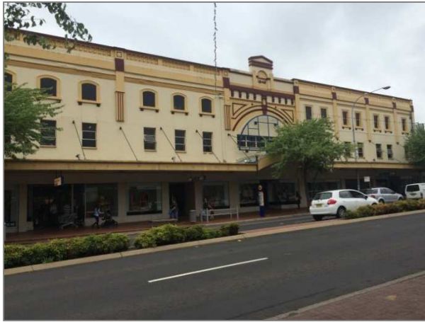
PICTURE 1 – SUMMER STREET FRONTAGE
