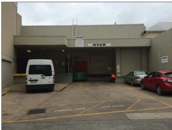
PICTURE 5 – SERVICE ENTRY
