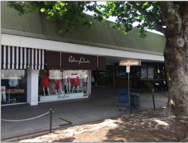
PICTURE 7 – ANSON STREET FRONTAGE
