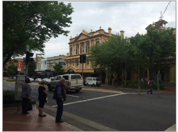
PICTURE 2 – SUMMER STREET FRONTAGE
